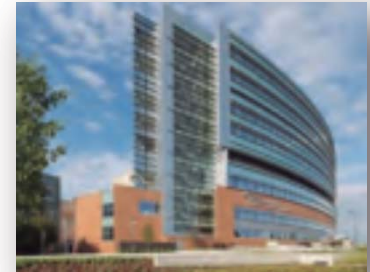
Lutheran General Hospital in Park Ridge, IL.
